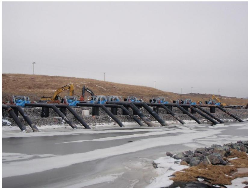
Photo 2-1: Newly Relocated Pumps with Suction Lines Installed at the Narrows
