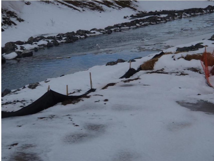
**Photo 4-1: Example of TP7 Environmental Controls Damaged by Winter Weather**
