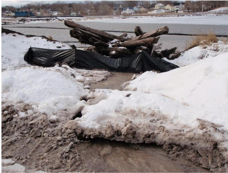
**Photo 2-4: Silt Fencing and Hay Bales Installed Along the East Access Road**
