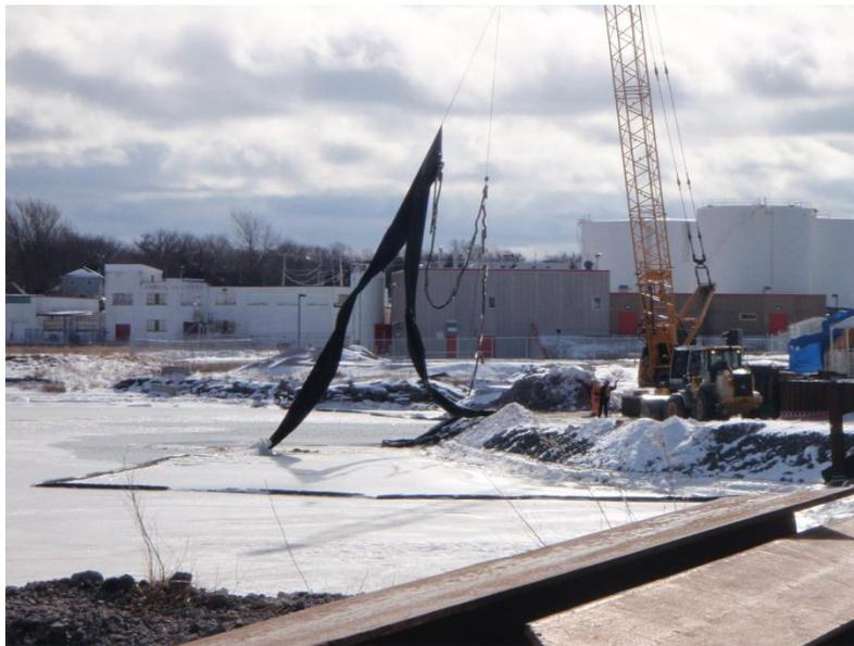
**Photo 2-3: Removing Derelict Silt Curtains from Battery Point Work Area**
