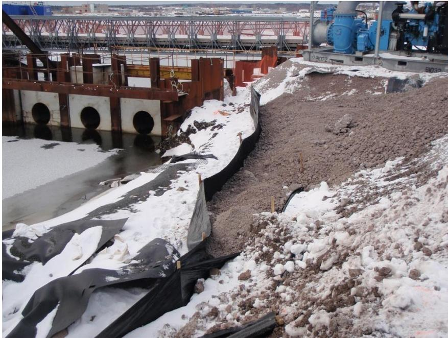
**Photo 2-2: New Silt Fencing along the Narrows Pump Pad**
