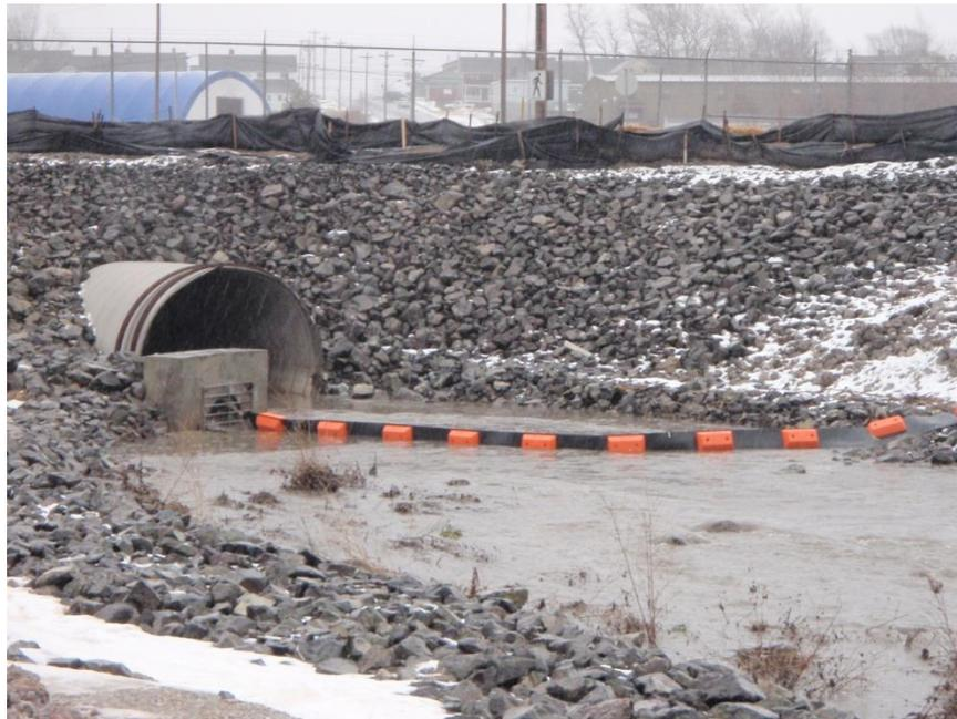
**Photo 2-3: New Debris Boom Downstream of Coke Ovens Brook Inglis St. Culvert**
