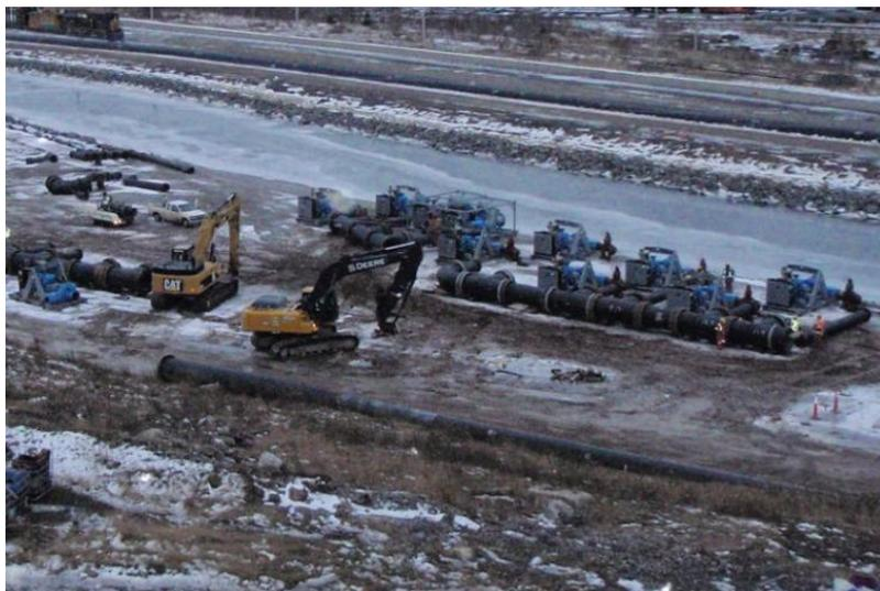
Photo 2-1: Relocation of Pumps from COB to the Narrows Dissipation Structure
