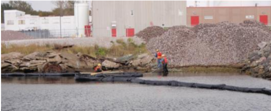
Photo 2-2: Silt Curtain Installation on West Side of Battery Point
