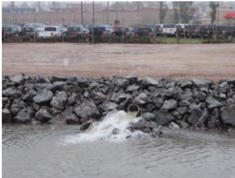
Photo 2-4: Turbid Water Discharging into the Main Channel via Outfall near Wash Brook
