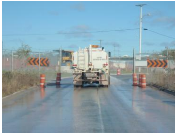
Photo 4-4: TP7 Water Truck Watering Ferry Street Access Road
