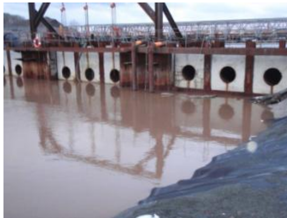
Photo 3-5: Pumping Over the Narrows Structure
