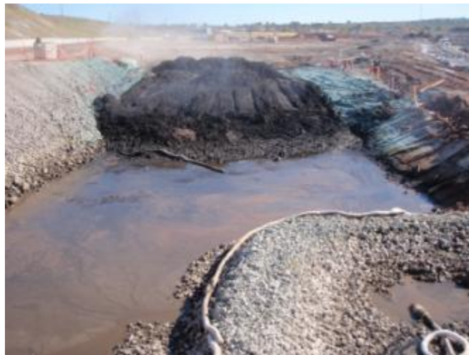
Photo 3-1: Dumping Impacted Material in the North Portion of the Northeast Sump
