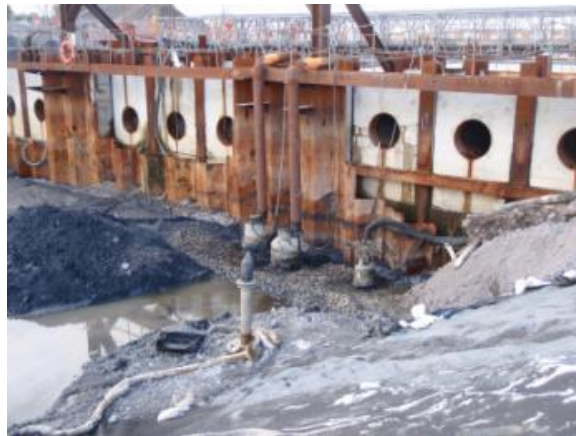
Photo 3-8: Rock Dams Constructed around Pumps at the Narrows
