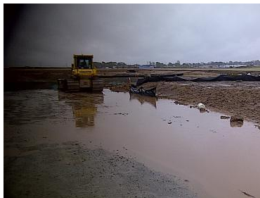
Photo 4-3: Phase I Clay Stockpile Silt Fencing Prior to Extension
