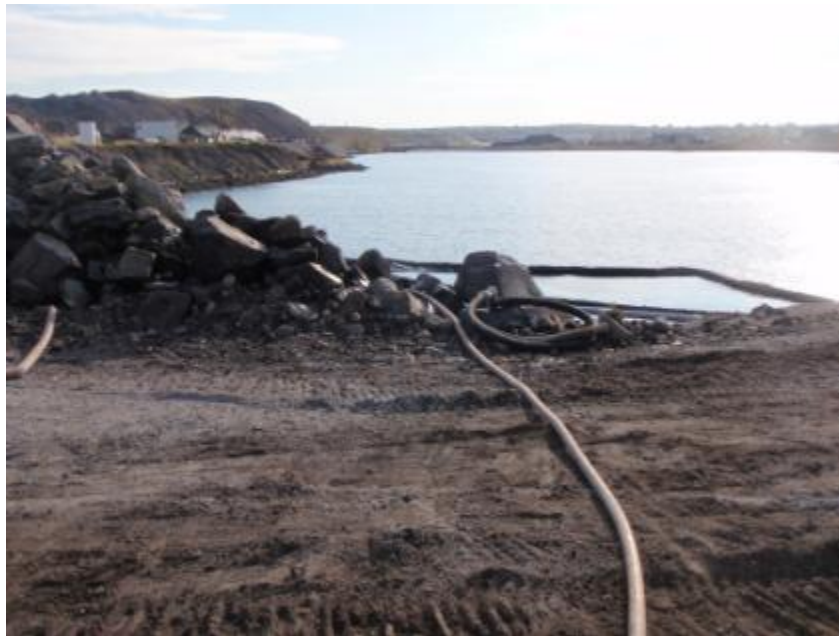
Photo 2-1: Decanting BPDS Cell into Northeast Corner of Phase III
