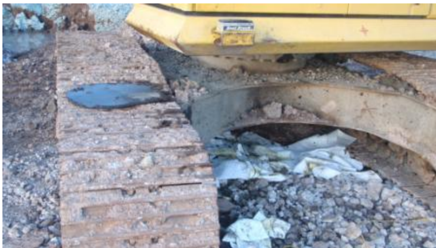
Photo 3-7: August 19, 2011 Hydraulic Fluid Leak
