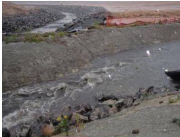
Photo 2-1: Turbid Water in Coke Ovens Brook Entering the Pumping Station
