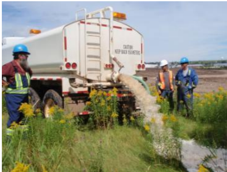
Photo 4-1: Discharging Clay Laden Water to the Former Landfill for Infiltration
