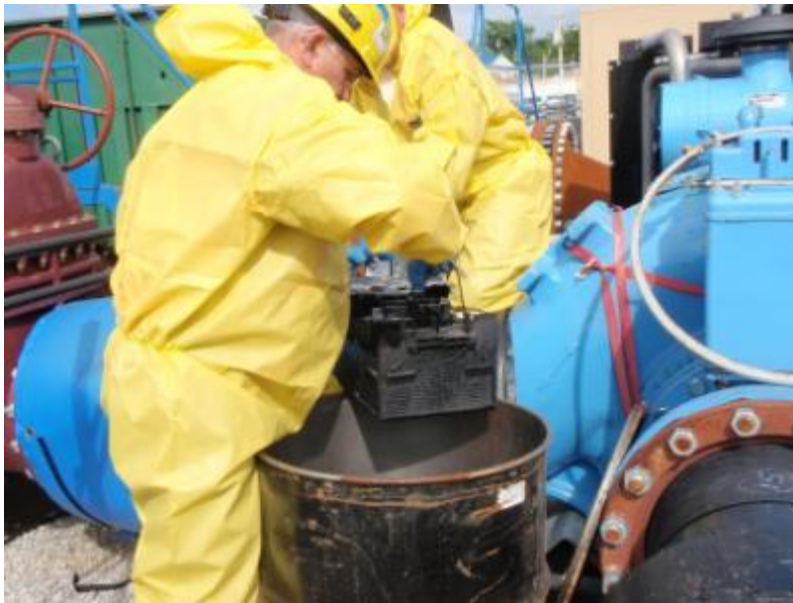
Photo 2-2: Removing Damaged Battery from Pumping Station
