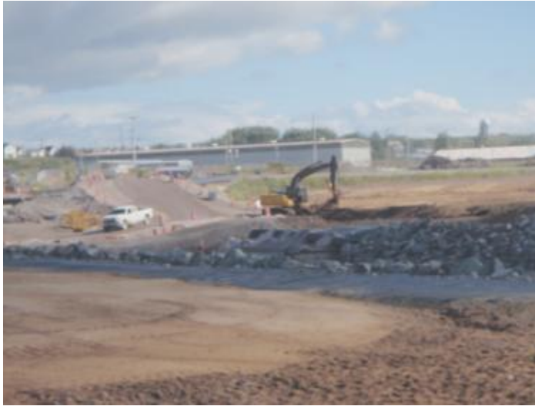
Photo 4-3: Reconstructing Berm near Phase I Access Ramp
